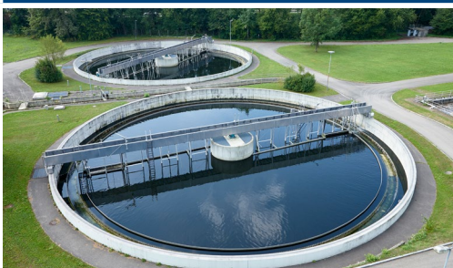
WATER & WASTEWATER P. 9
